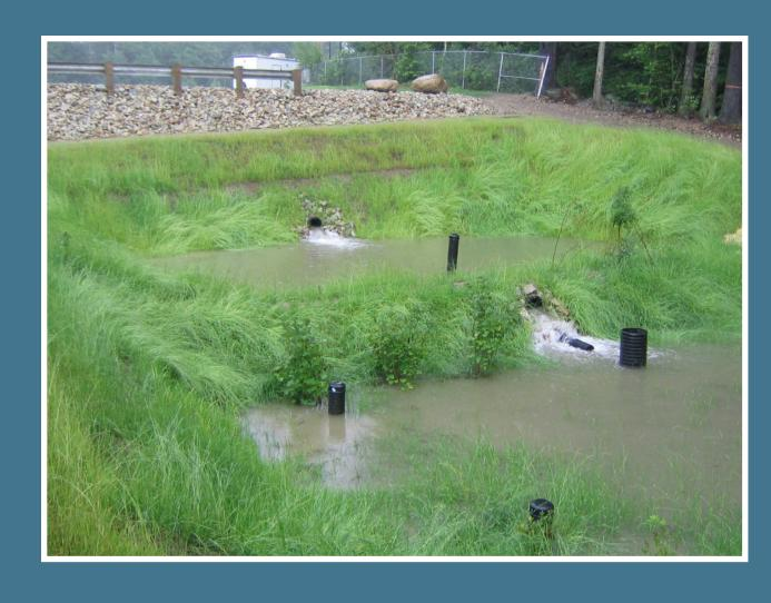
A recent innovation in stormwater design, the subsurface gravel wetland looks and functions like a natural wetland, effectively removing sediments and other pollutants found in runoff, while enhancing the landscape's visual appeal. Unlike other stormwater wetlands that function more like ponds, this wetland relies on a dense root mat, crushed stone, and a microbe rich environment to treat water quality.
